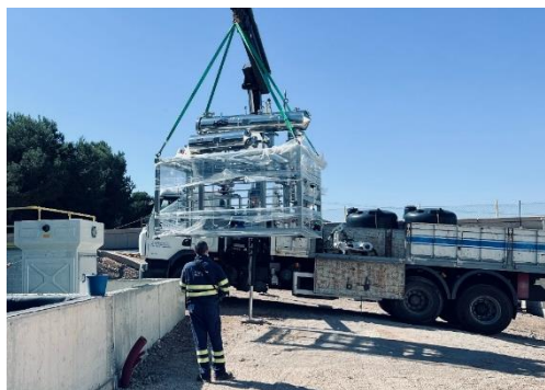
Figure 3. Installation of the MVC equipment. LIFE-Desirows project (Cartagena, Spain)
