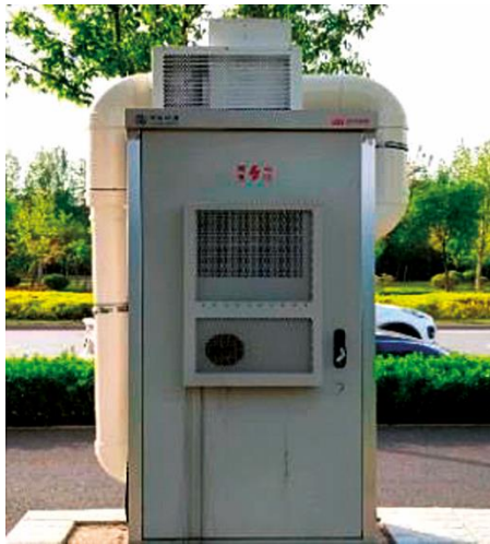
Figure 2. Installation of an energy-saving integrated thermal management system
