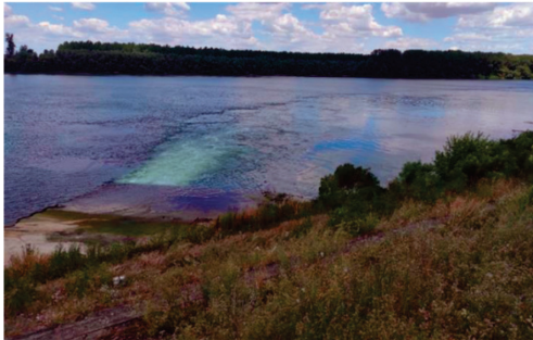
Figure 4. Realistic representation of the inflow channel and the Sava River at the thermal power plant Nikola Tesla B
