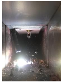
(b) Sprinkler heads without HCP
