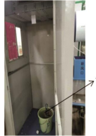
Figure 6. Test bench for natural cooling
