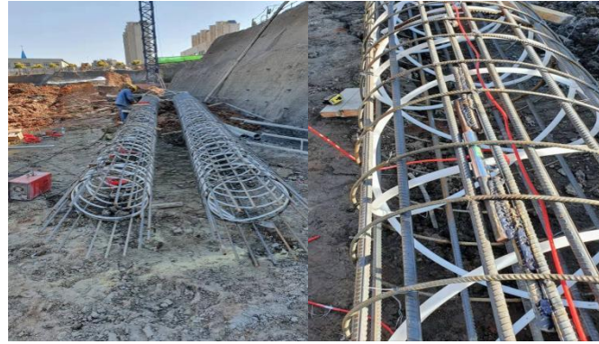
(a) Layout of the steel bar cage (b) Sensor installation
