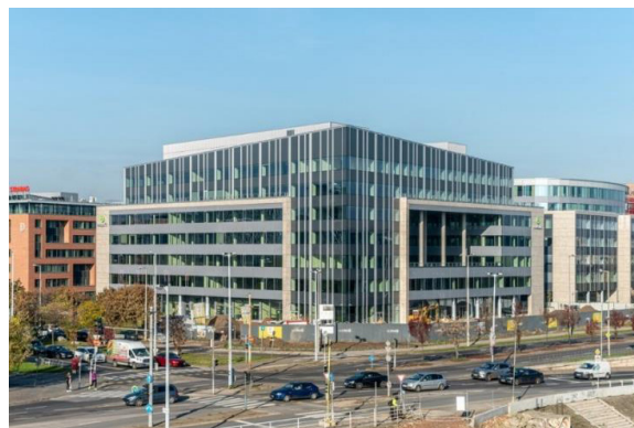
Figure 2. Innovation Campus office building [27]
