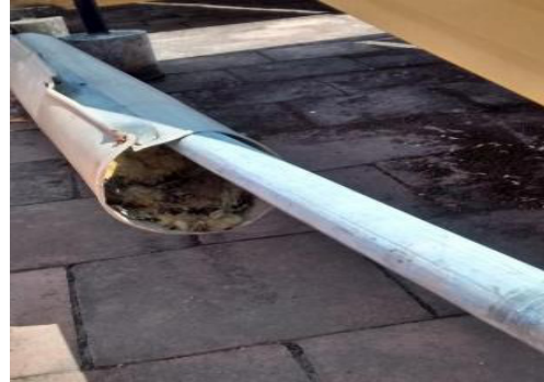
Figure 4. Insulation of pipes using glass wool
