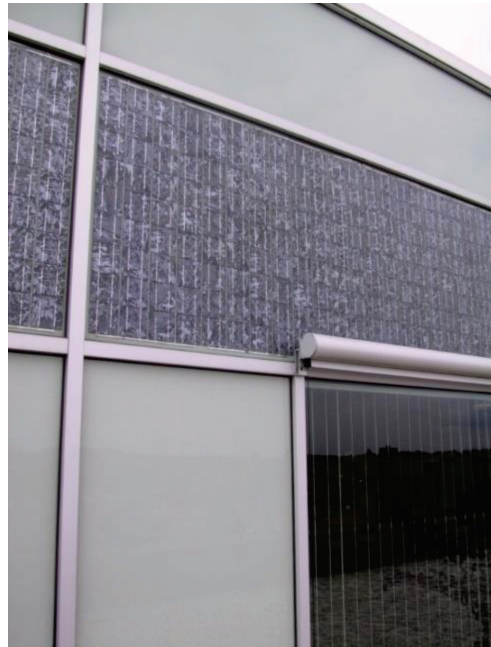
Figure 20. Exterior shading blinds installed during building renovation not considering the shading of the adjacent BIPV modules
