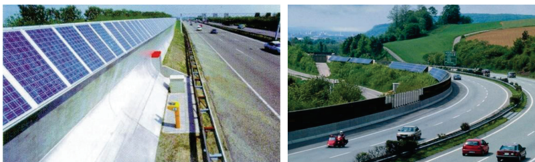
Figure 7. The PV sound barriers
