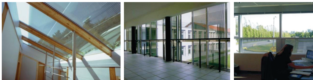
Figure 6. The PV windows
