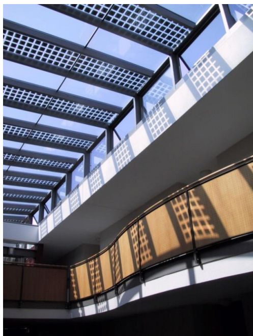
Figure 18. The BIPV skylight comprising an alternating pattern of glass and BIPV modules
