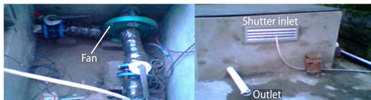
Figure 6. The room for inducing and exhausting air of soil-air heat exchanger
