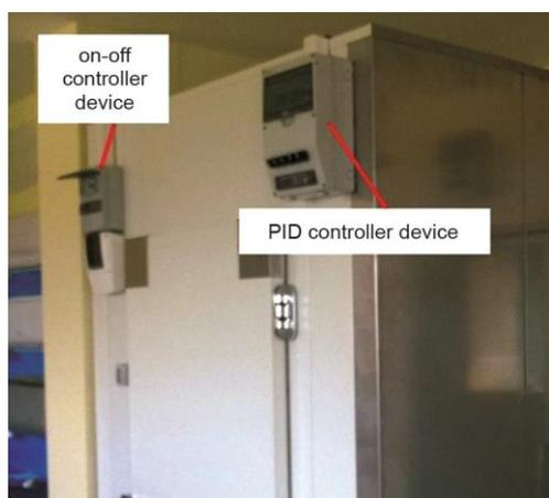
**Figure 3. The position of the controllers**
