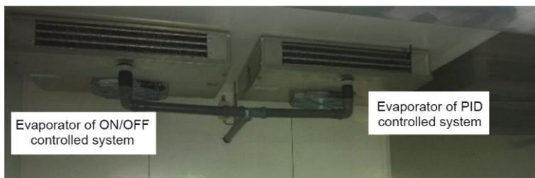
**Figure 2. The position of the evaporators in the chamber**
