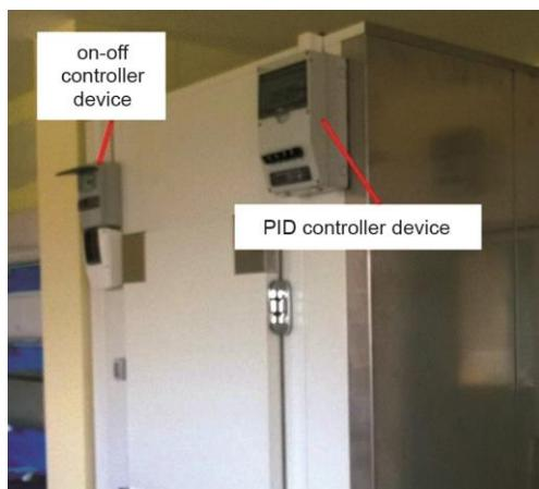
Figure 3. The position of the controllers
