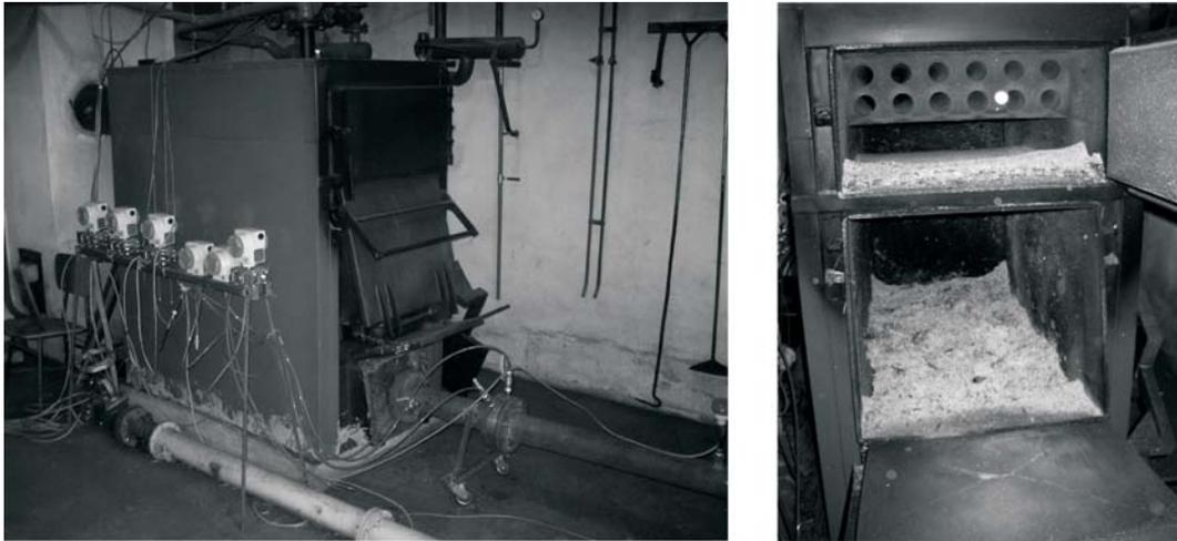
**Figure 2.** The hot water boiler at the time of research with functional parts: ash collector, furnace, secondary combustion chamber, and the flue gas tube
