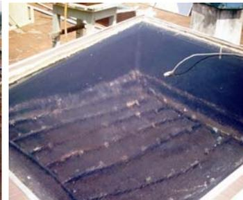
**Figure 3. Photograph of the dripping arrangement with black sponge liner**
