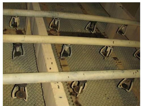
Figure 5. Nozzles and fill packing
