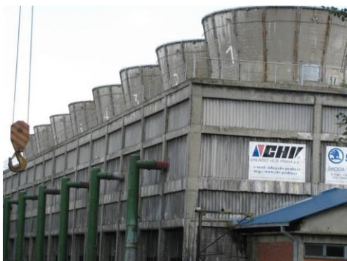
Figure 4. Cooling towers of the power plant
