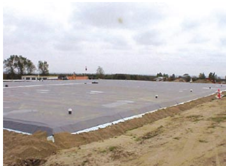
Figure 6. Pit heat storage
