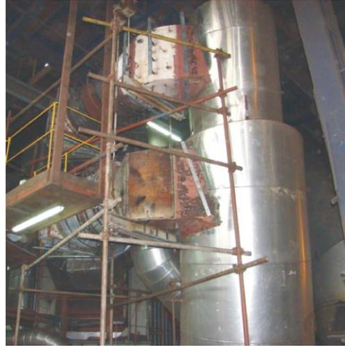
**Figure 3. Place on the lower channel of the mill No. 3, which was repaired after damage**
