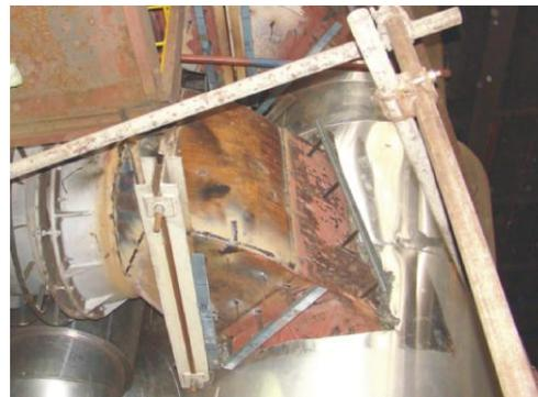
**Figure 5. Lower channel elbow repaired after damage**
