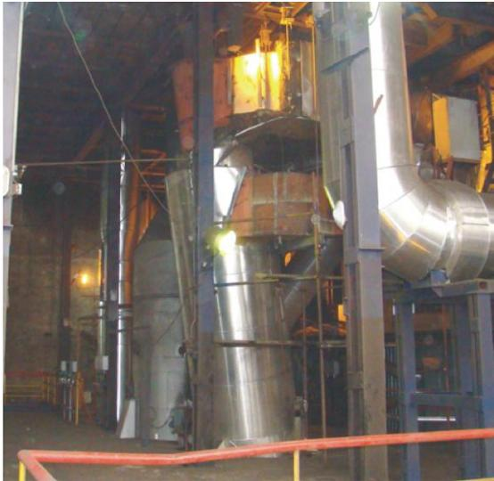
**Figure 2. Photo of aero-mixture splitter and both horizontal channels**
