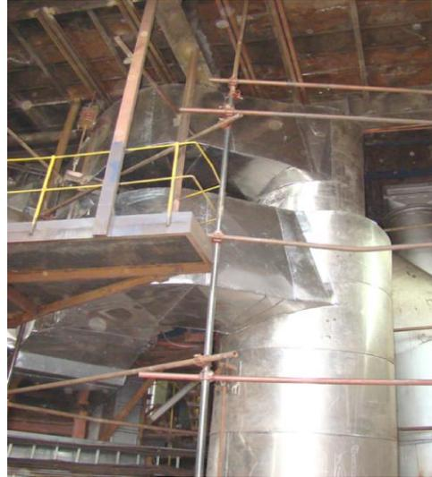
**Figure 12. Reconstructed channel – connection with aero-mixture splitter**
