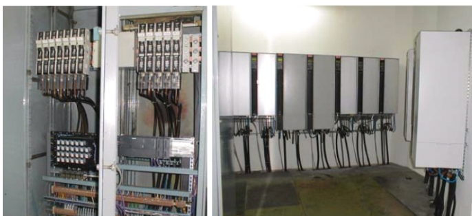
Figure 11. Substation and control system (left side), converters (right side)
