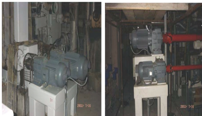
Figure 13. Driving motors of the new drive, directly coupled (left side), or across cardan shaft (right side)
