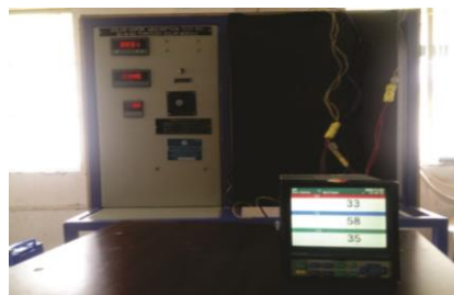
Figure 5. Refrigerator placed indoor
