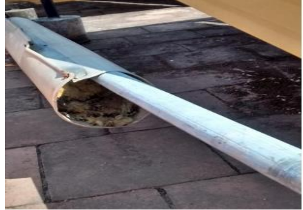
Figure 4. Insulation of pipes using Glass wool
