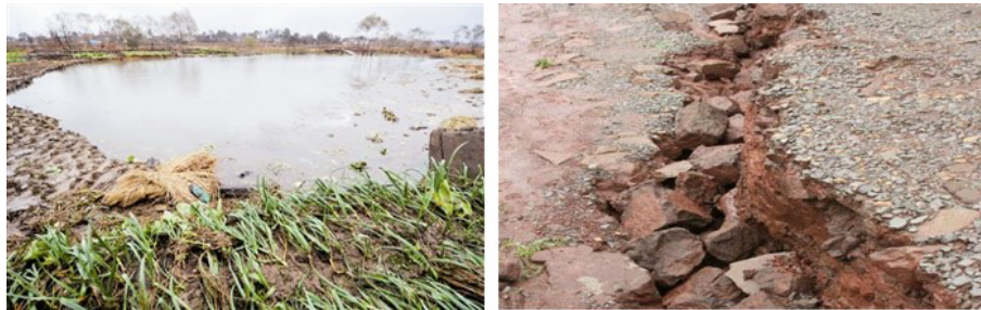
Figure 1. Typical salt mine ground subsidence hazards
