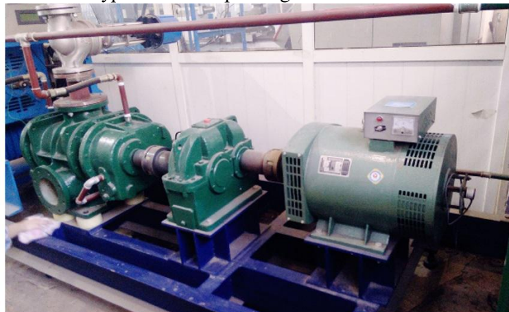
Fig. 9 Test platform for power module of Roots-type waste heat power generation device
