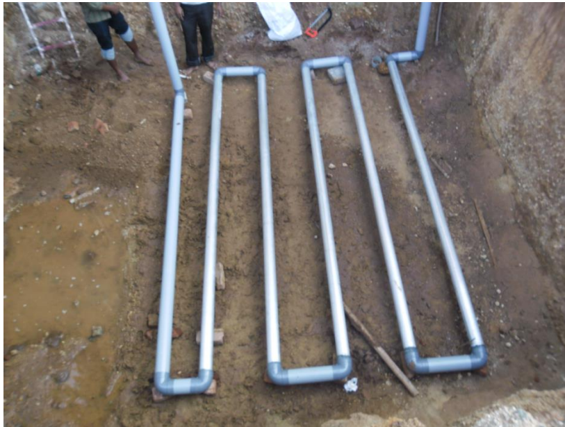
Figure 2. Underground pipe in SAHE system
