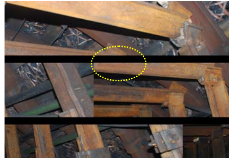
Figure 17. Connecting parts of U-shaped steel support
