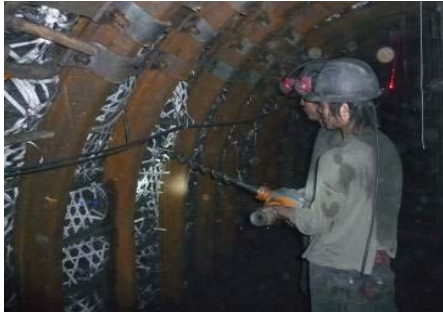
Figure 14. Miners drilling the pressure-relief hol
