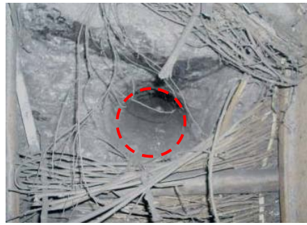
Figure 15. A pressure-relief hole
