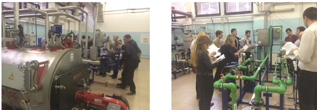
Figure 5. Implementation of exercises boiler plant with condensate drainage system and pump plant in the Laboratory for practical training of energy managers
