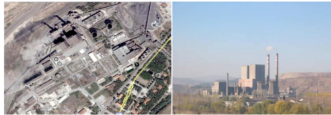
Figure 1. View of the thermal power plant site
