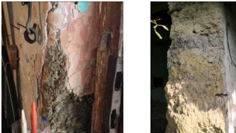
Figure 3. Rammed earth wall with a large quantity of added straw (chaff) plastered with mud mortar, a house in Vojlovica.
