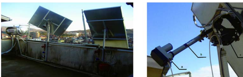
Figure 2. Experimental set-up and a segment of the tracking system: electric drive (a); gear spindle (b); auxiliary mechanism (c)
