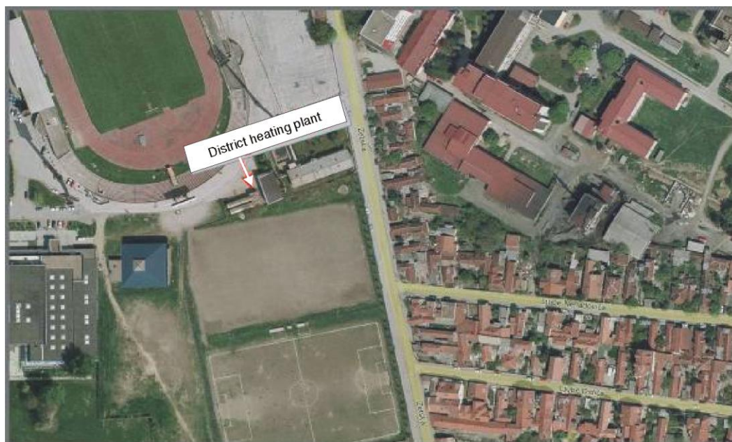
Figure 26. Public utility company – district heating plant “Čair”
