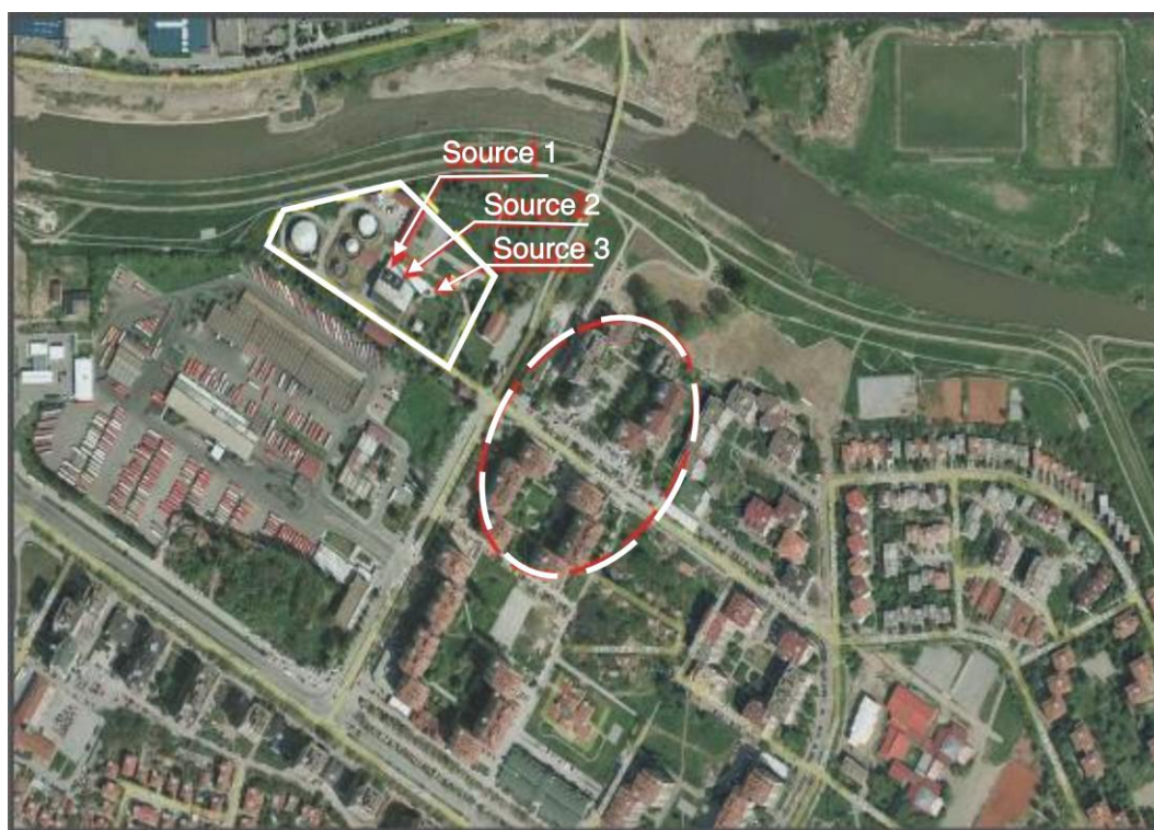
Figure 1. District heating plant “Krivi vir” (full white boundary), its heat source and the surrounding residential area (dashed white boundary)
