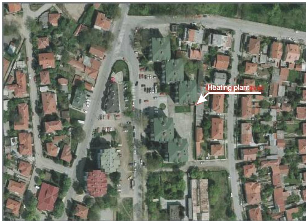
Figure 16. Public district heating utility company “Pantelej” and its heating source
