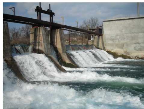
Figure 6. The photo of constructed MHPS, existing weir, and added logs
